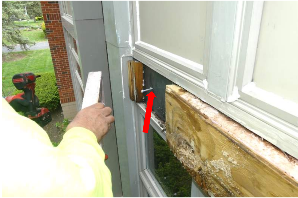
Photo 27 – Screw through insulation
