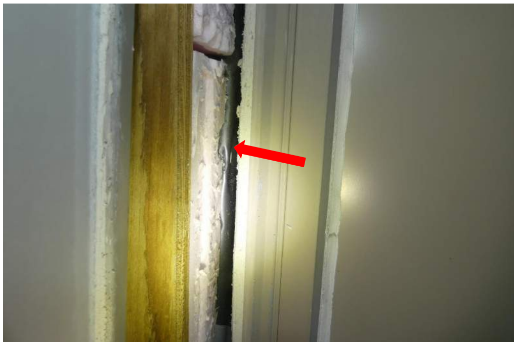
Photo 34 – Flashing membrane behind insulation
