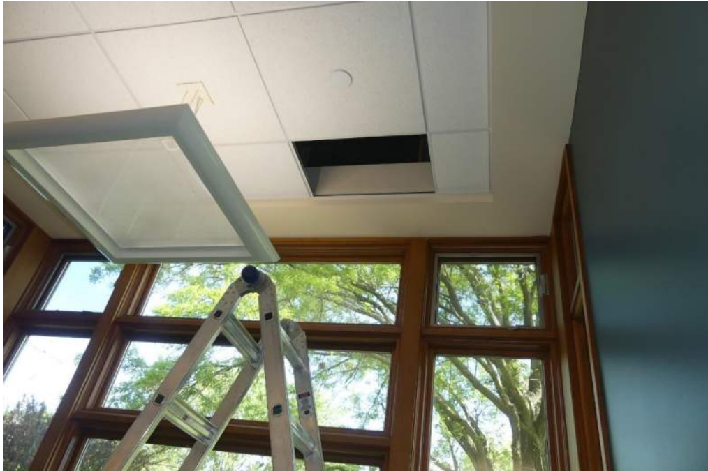
Photo 11 – Ceiling tile removed at middle bay
