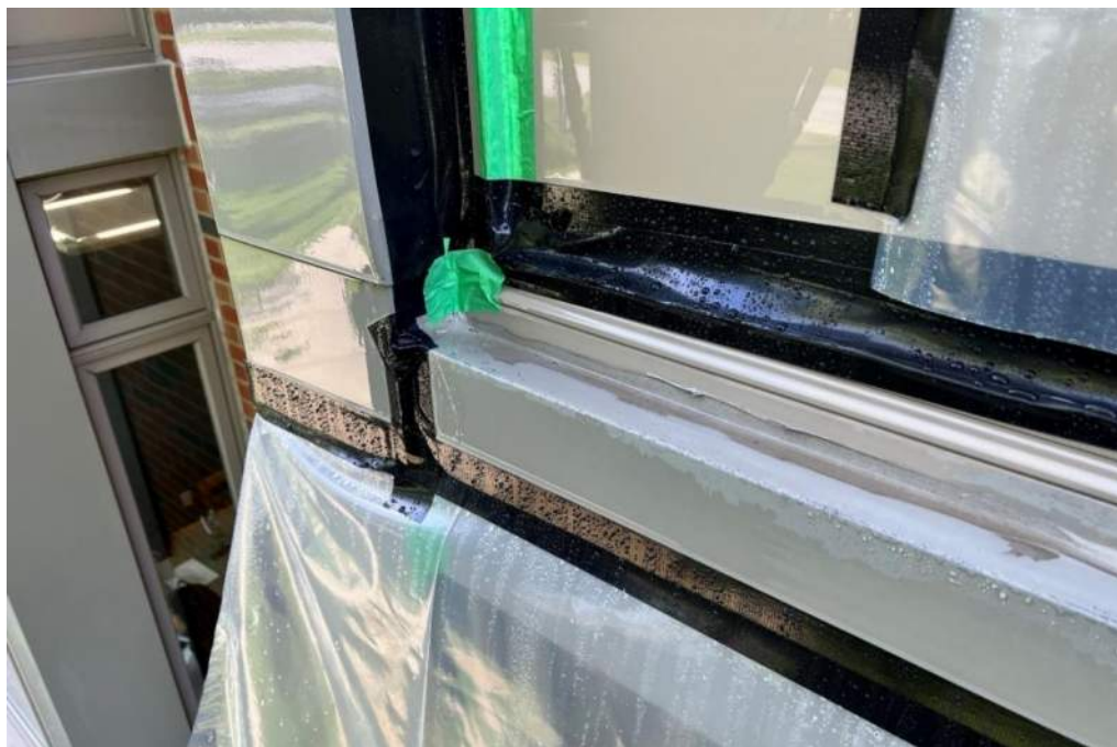
Photo 18 – Masking of various components
